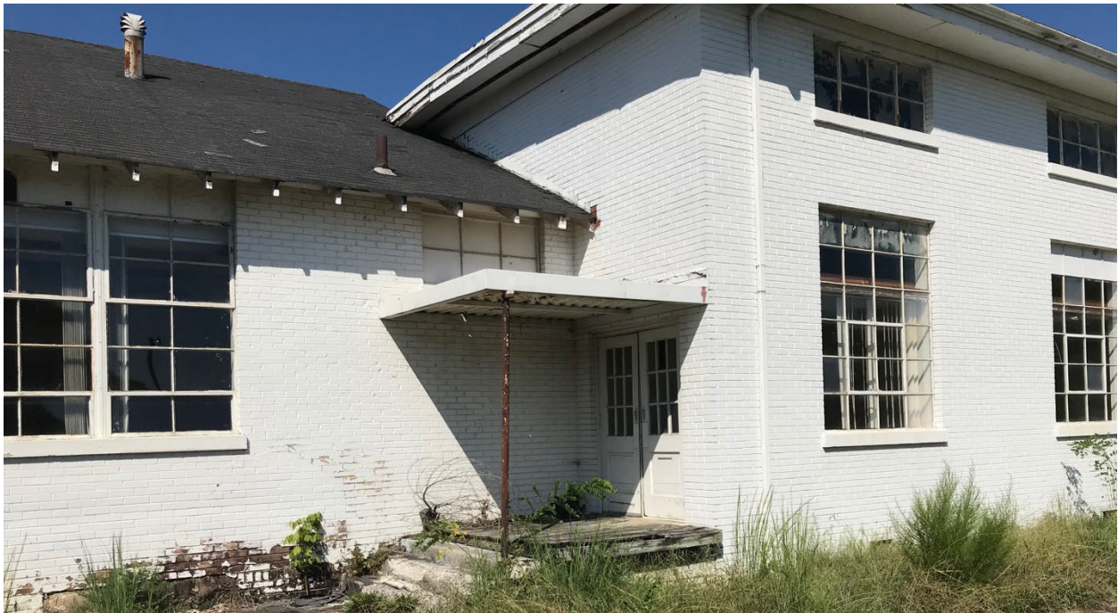
Primary entrance into the gymnasium, note original double doors and extant windows. Concrete steps have deteriorated.
