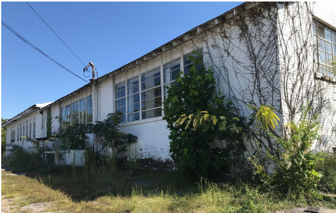
West elevation, emphasizing 1937-1938 section. Note that rafters and windows are intact. also note problem with foliage and moss/weeds around A/C unit.
