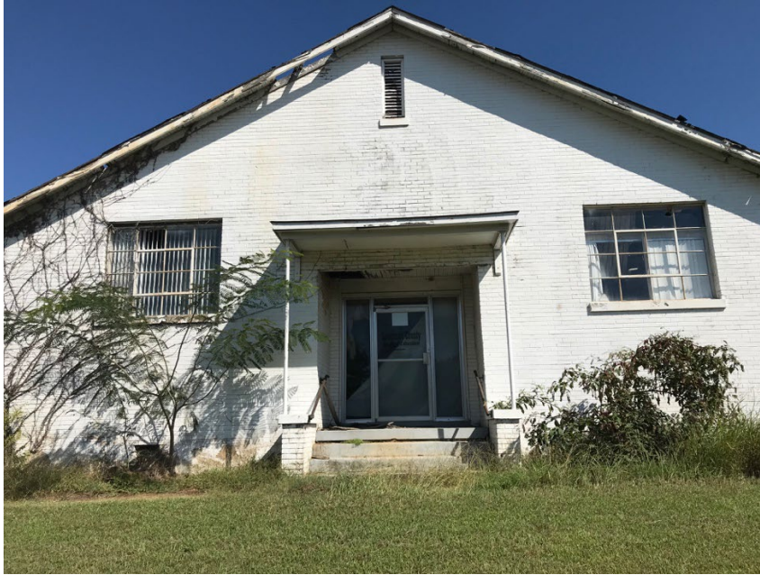
South entrance. Note intact windows, roof damage, and excess foliage along the walls.
